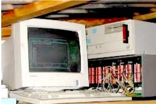
Located in the roof of the test room - Data Collection, Recording and Control.
